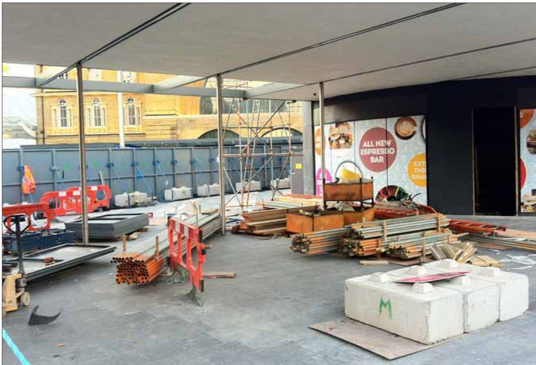
Figure 4. Construction in Granary Square (October 2013).
