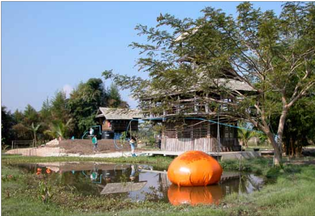
Figure 5. The SUPERFLEX's Supergas Biogas System. Photograph provided by the artists of the The Land Foundation.
