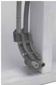
Stacked PEX Elbows, mounted to stud
